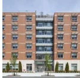
THE CONCERN HEIGHTS APARTMENTS
